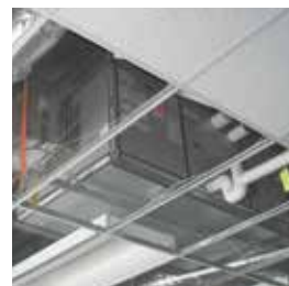
Suspension rods eliminate need for support brackets
