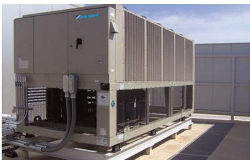
Trailblazer chillers utilize environmentally responsible R-410A refrigerant and meet or exceed the performance requirements of ASHRAE 90.1 2013. Industry leading part load efficiency is obtained through the use of variable speed condenser fan technology. High overall efficiency = lower annual energy costs.
