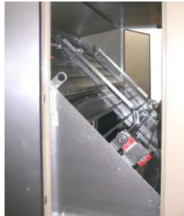
Standard low-leak dampers for superior resistance to air leakage and reduced energy costs.
